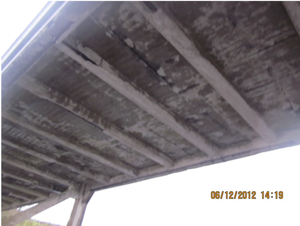
Photograph 9: Soffit, exposed reinforcement.
