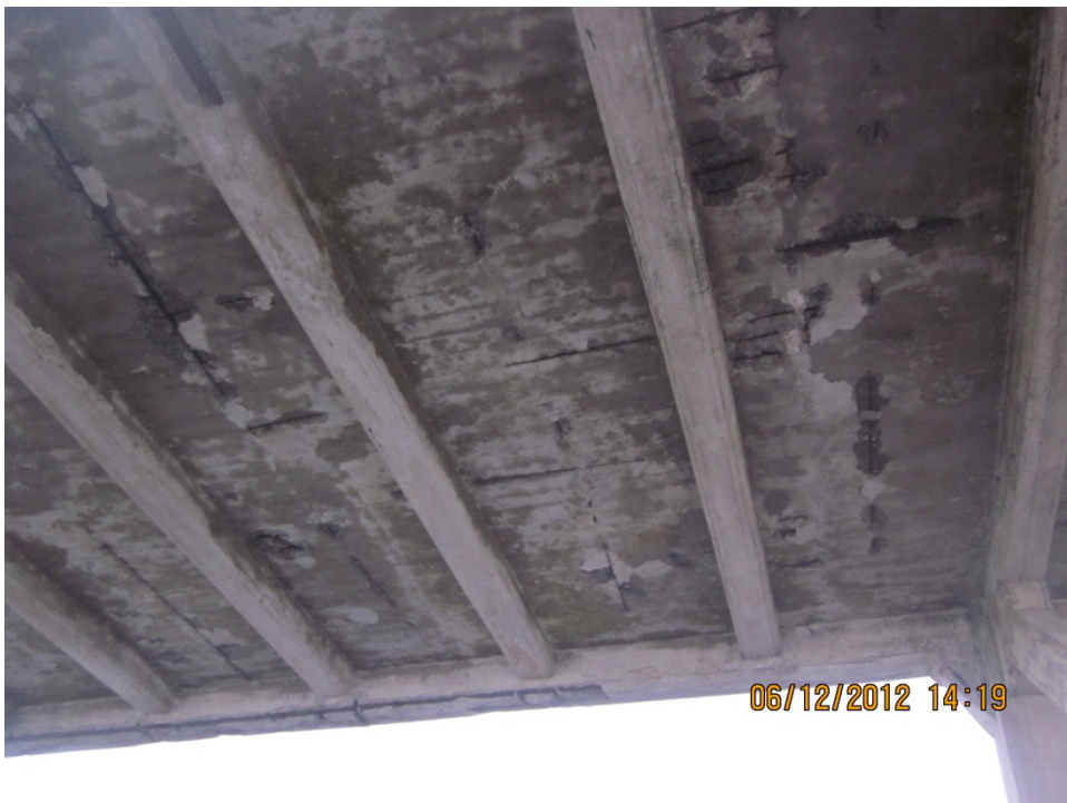
Photograph 8: Soffit showing spalling.
