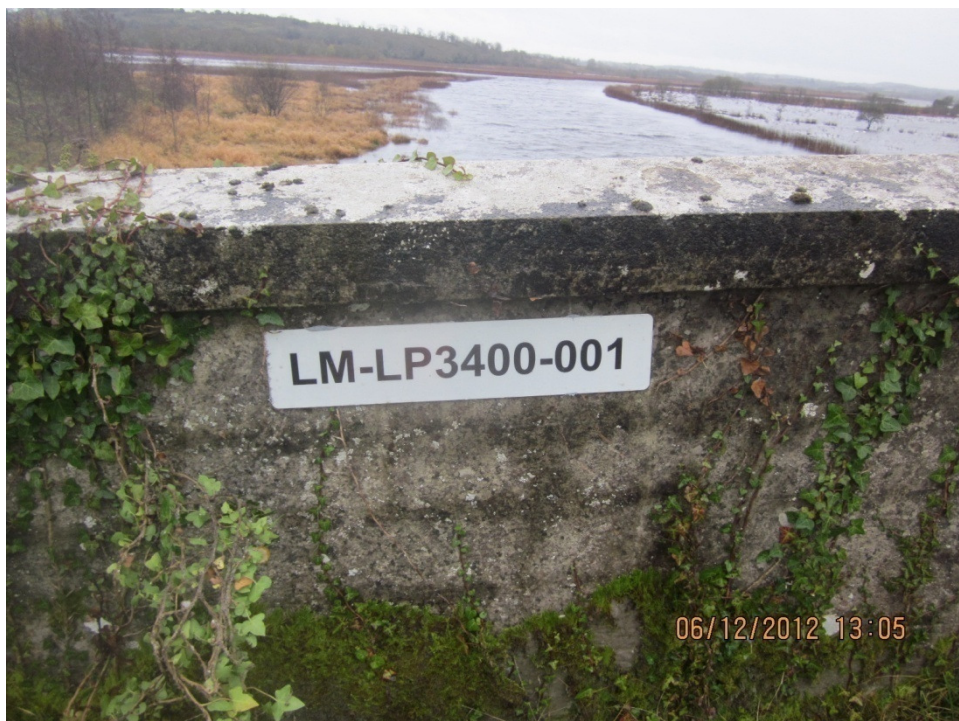
Photograph 2: Parapet with bridge reference plate.
