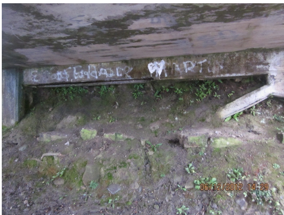
Photograph 4: West side abutment with earth revetment.
