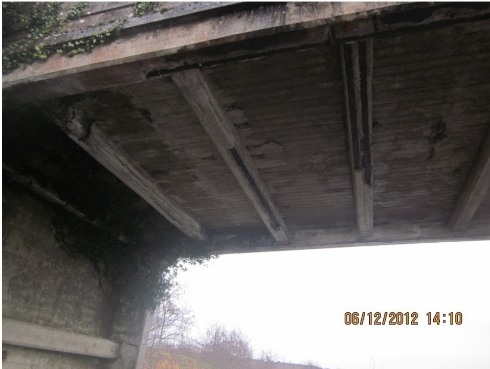
Photograph 7: Soffit showing spalled concrete and exposed rebar.
