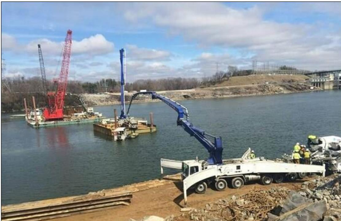
*Plate 2-1 Example of concrete pour across river to piled cofferdam*
