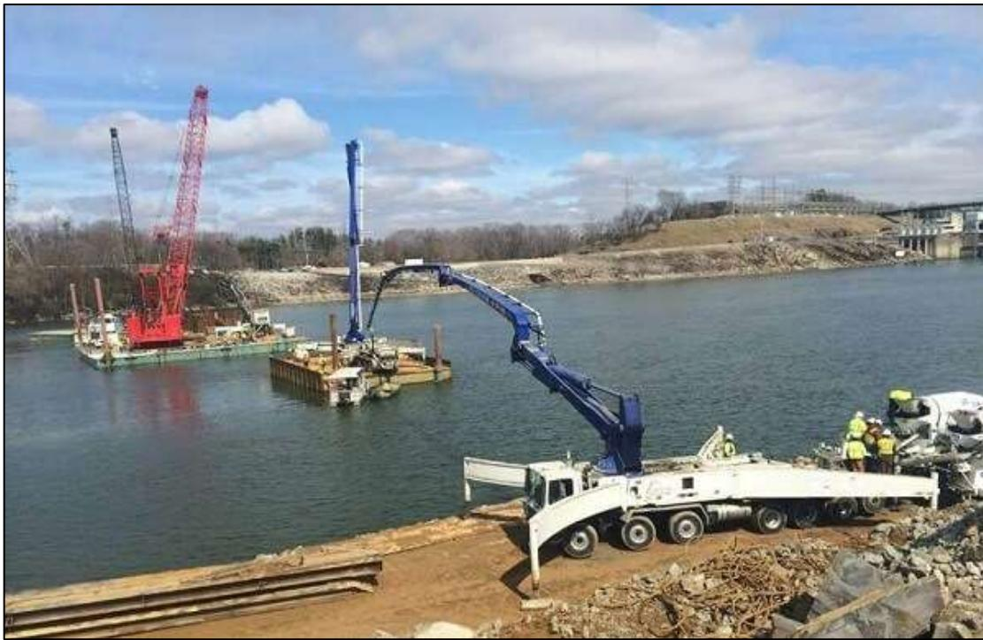
Plate 3-1 Example of concrete pouring taking place across a river
