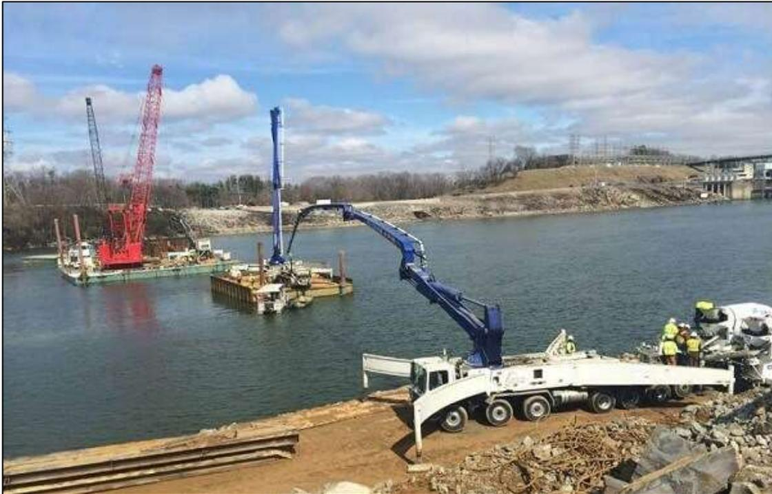
Plate 2-1 Example of concrete pouring taking place across a river
