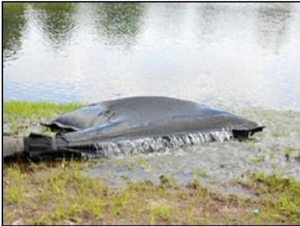
Plate 3-2 Silt bag typical use no. 2
