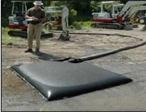
Plate 3-1 Silt bag typical use no. 1
