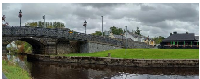
View of Leitrim Bridge during a site walkover in September 2024.
