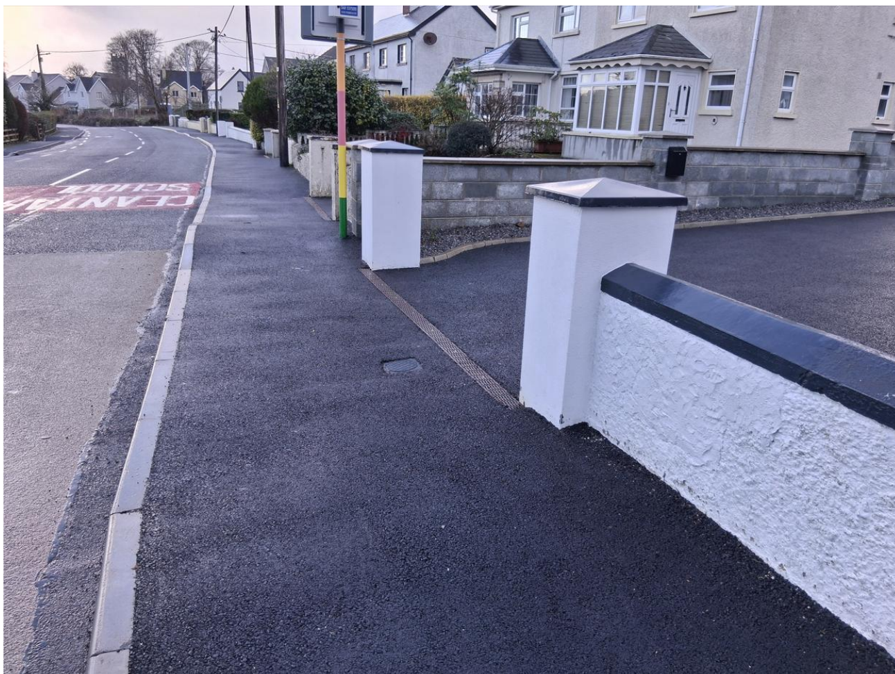
Churchfield, Dromahair – Provision of new Footpath under an Active Travel Scheme
