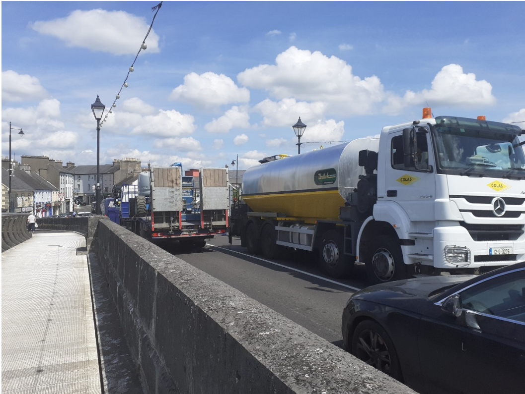
Plate 2.7.6 Existing River Shannon Bridge, Carrick-on-Shannon
