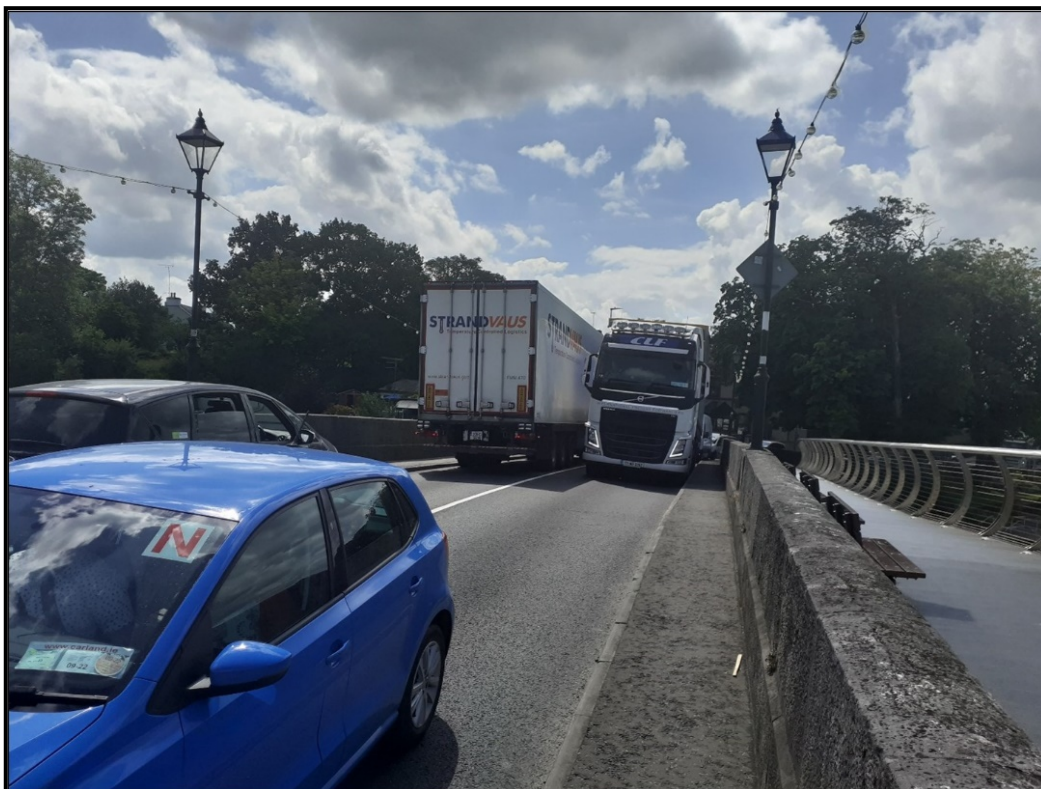
Plate 2.7.5 Existing River Shannon Bridge, Carrick-on-Shannon
