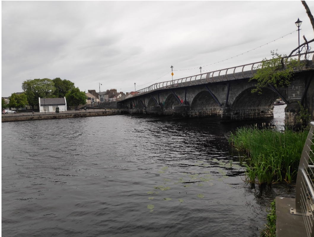
Plate 8.5.6 River Shannon Pedestrian Bridge
