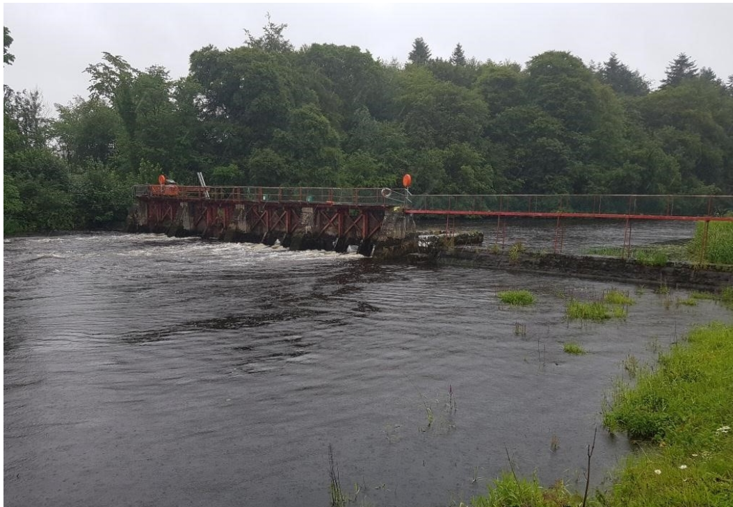
Plate 4.13.4 Summer Operation at Jamestown Weir with Levels Low and Not Discharging over the Permanent Weir Section
