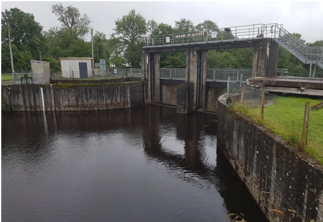
Plate 4.13.2 Lough Allen Controlled Outflow at Bellantra Sluices
