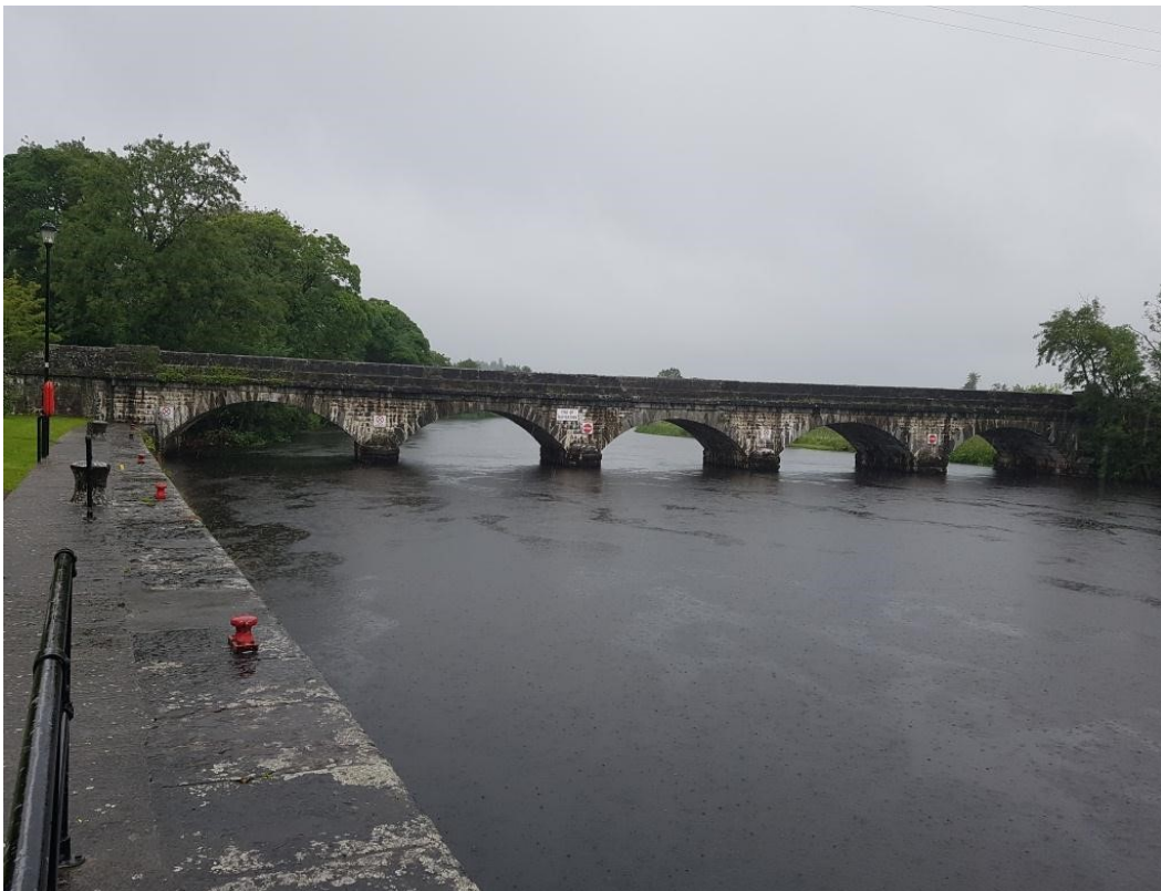
Plate 4.13.6 Jamestown Bridge Crossing
