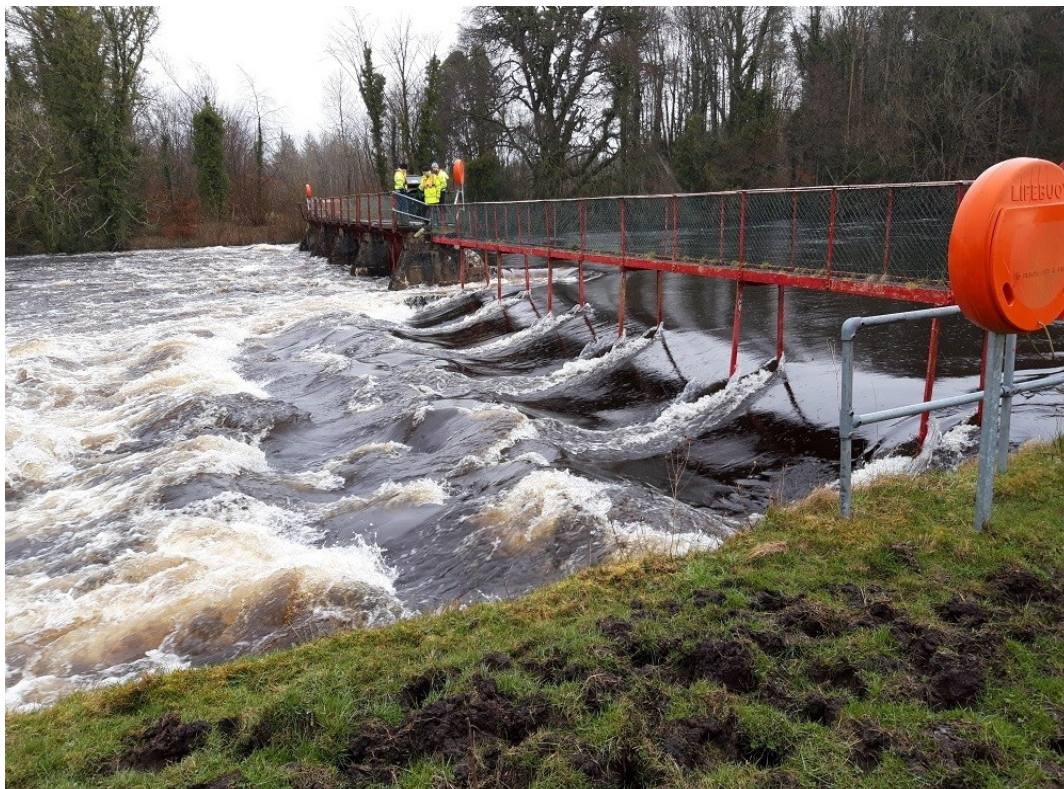
Plate 4.13.3 View from Jamestown Weir (taken 27 February 2020) (note all flow at that time within channel and discharging over the Permanent Weir Section also)
