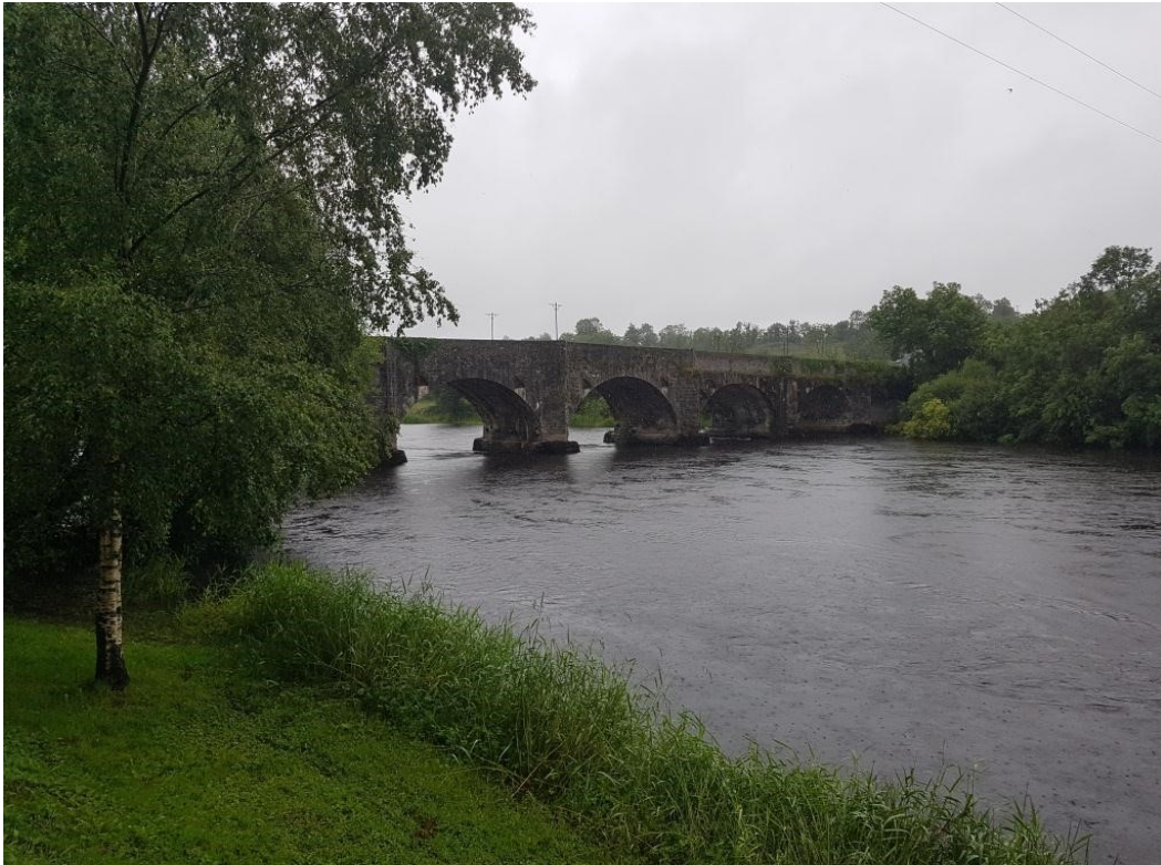
Plate 4.13.7 Drumsna Bridge Crossing
