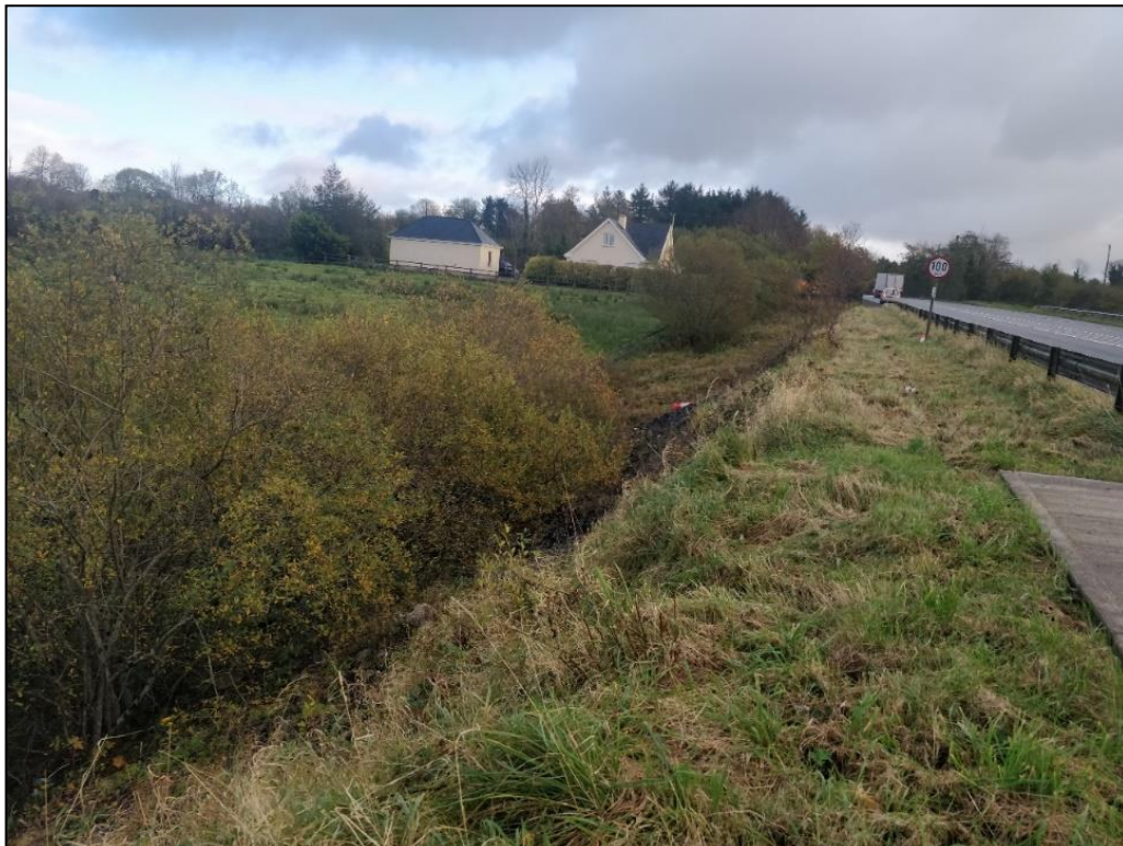
L15.3 Existing N4 embankment looking towards Aghamore on the left hand side of the road (eastern side)
