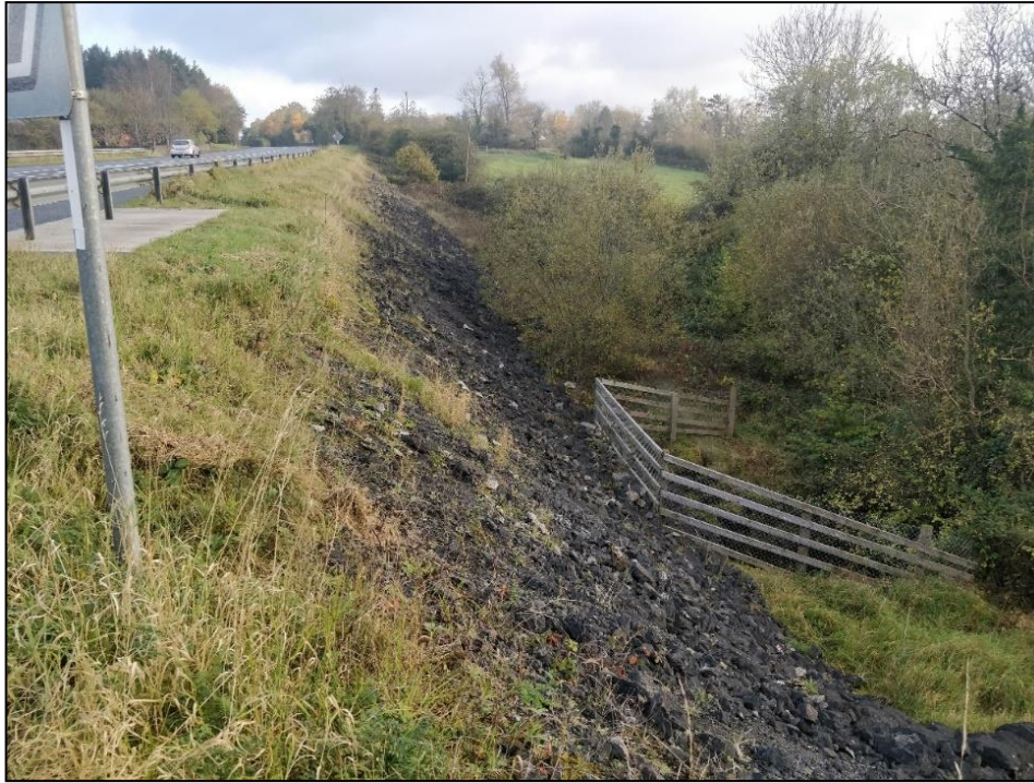
L15.2 Existing N4 embankment looking towards Aghamore on the left-hand side of the road (eastern side)
