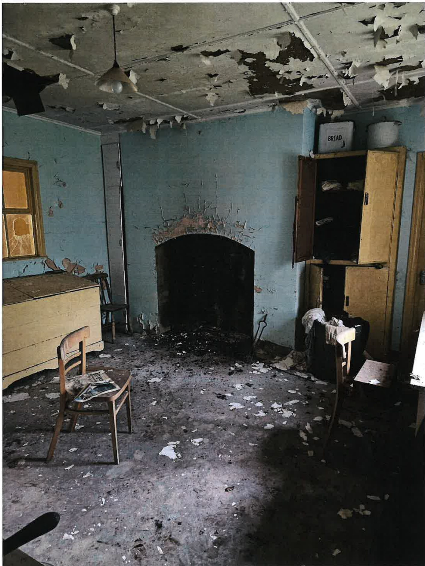
Photograph no. 7 is the living room.
