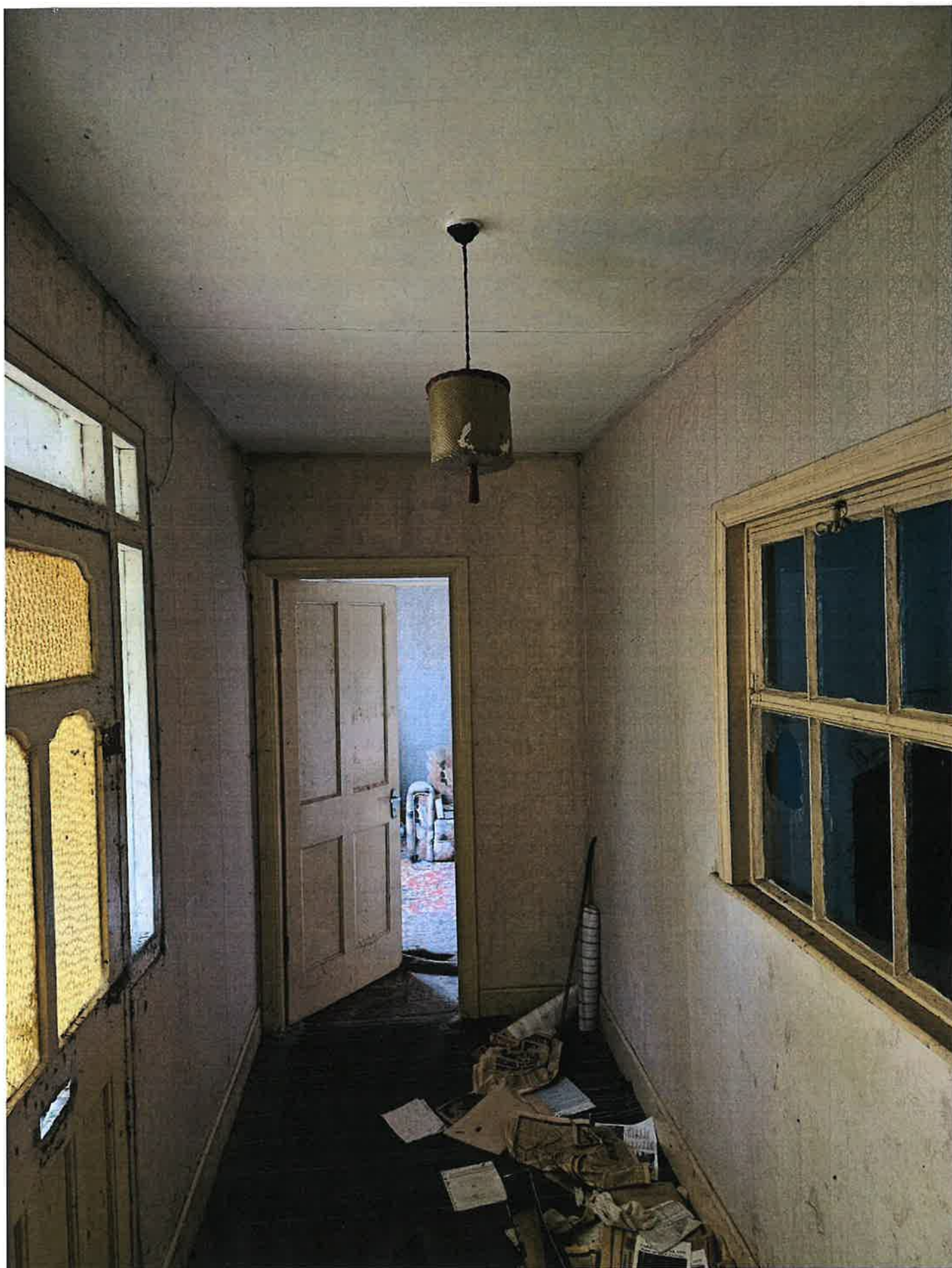
Photograph no. 3 An internal view of the entrance hall.
