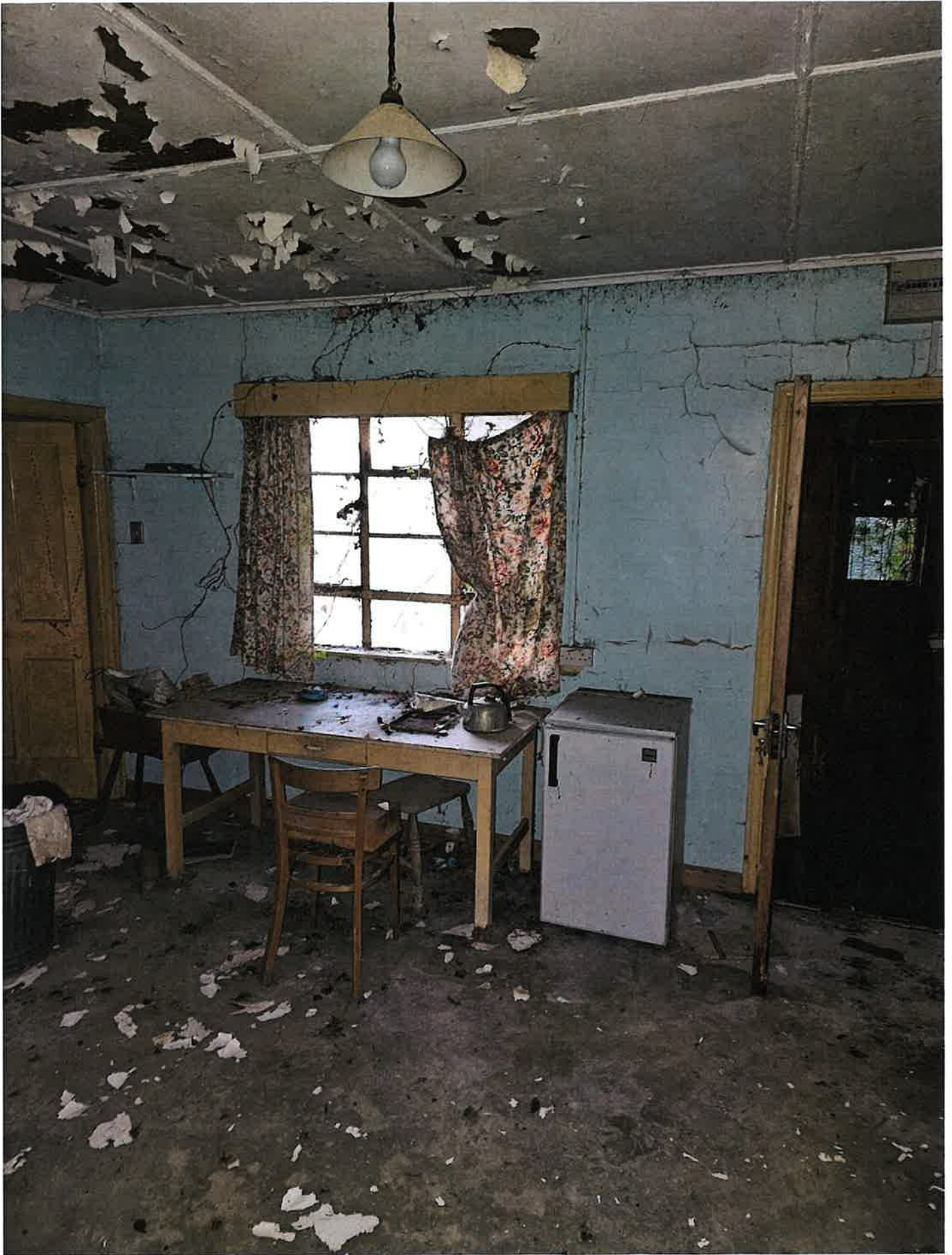
Photograph no. 8 is a view of the rear wall of the house from inside the living room. The opening to the proposed extension will be through the existing window opening, which will be removed and the opening adjusted as part of the works
