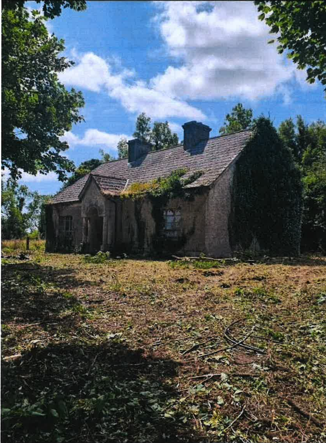
Photograph no. 2 Taken July 2026 showing the front and side elevation
