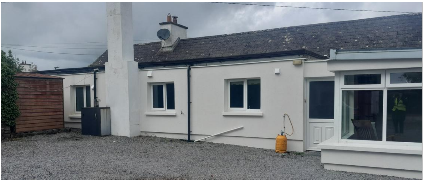
Fig.1 – Rear elevation of dwelling with conservatory on RHS
