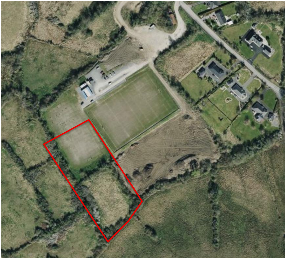
Figure 3: Approximate extent of works relative to existing playing pitch and adjoining dwellings
