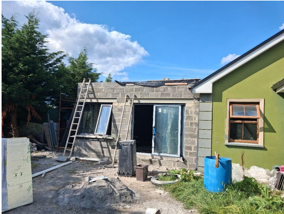
Fig. 3 – Image of rear of subject dwelling, where the extension is currently under construction.
