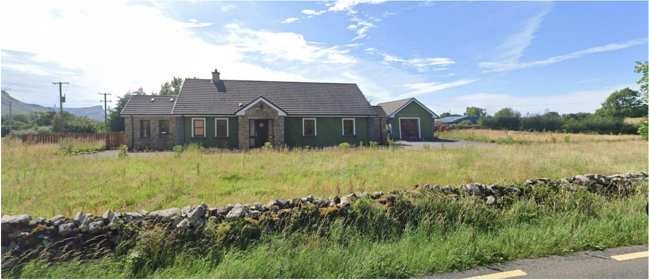
Fig.1 Front elevation of existing dwelling
