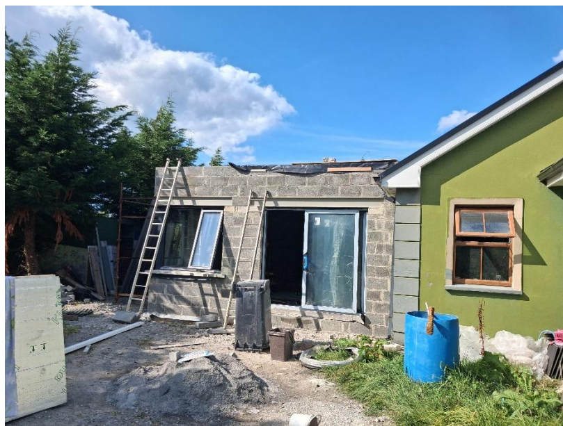
Fig.6 Subject extension under construction
