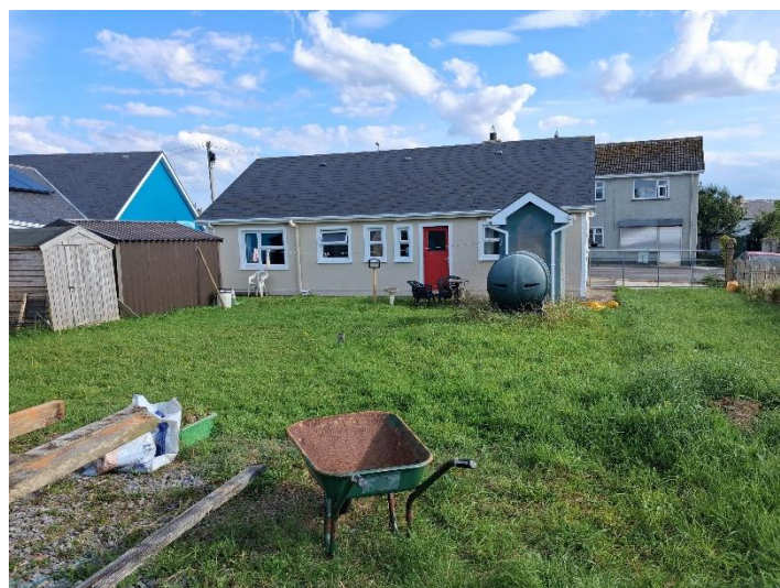
Fig. 3 – Rear of subject dwelling
