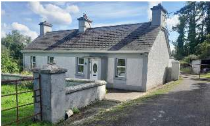
Fig. 2 – Existing dwelling (front)
