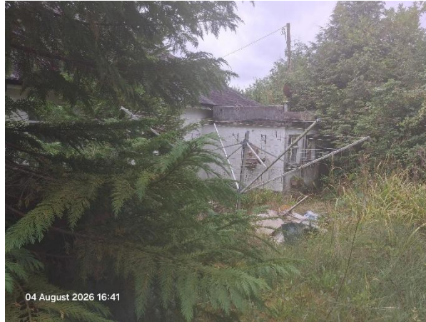
Fig. 3. Rear of the property
