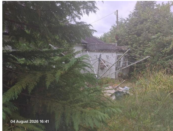
Fig. 1. Rear of the property showing as built extension
