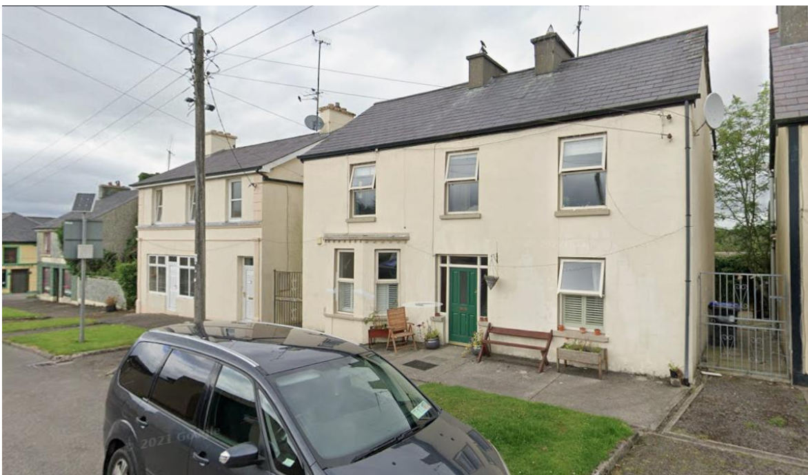
Fig. 2 Two storey dwelling on site.
