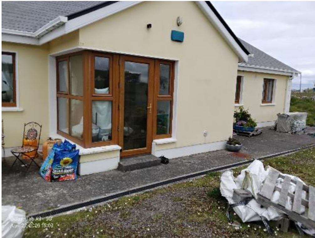
Fig. 3– Image of rear of subject dwelling, where proposed extension is to be located.
