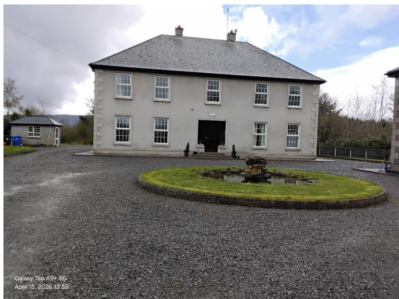
Fig. 2 Two storey dwelling on site.
