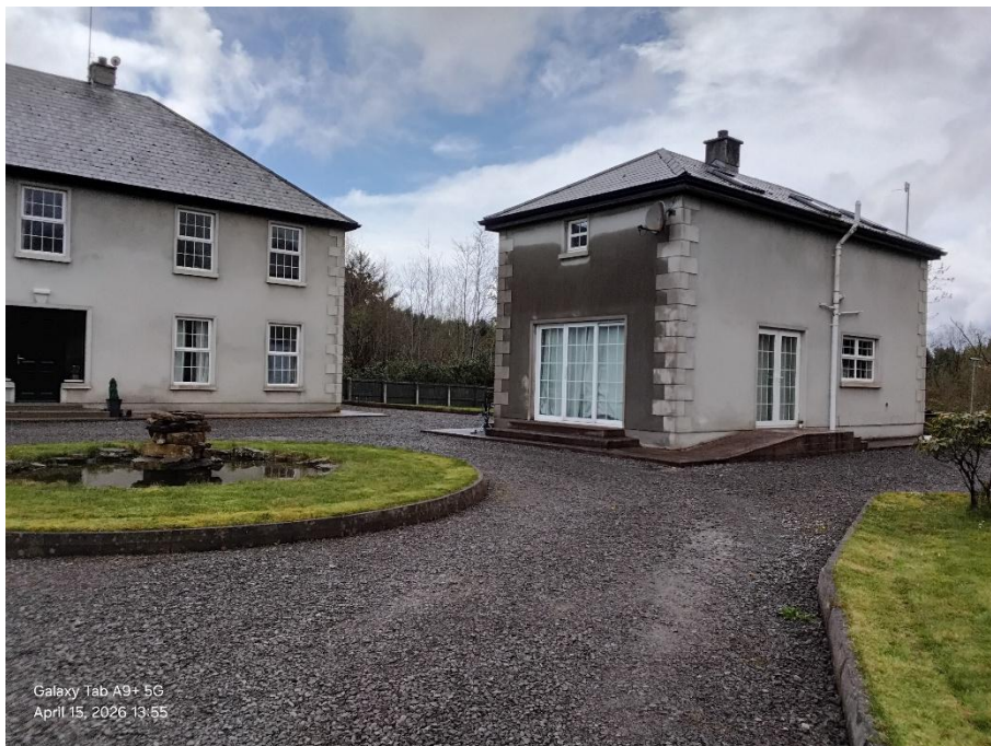
Fig. 3 Location of both structures on site.
