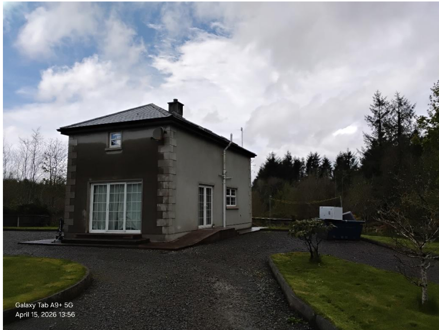
Fig. 3 Two storey garage structure on site.
