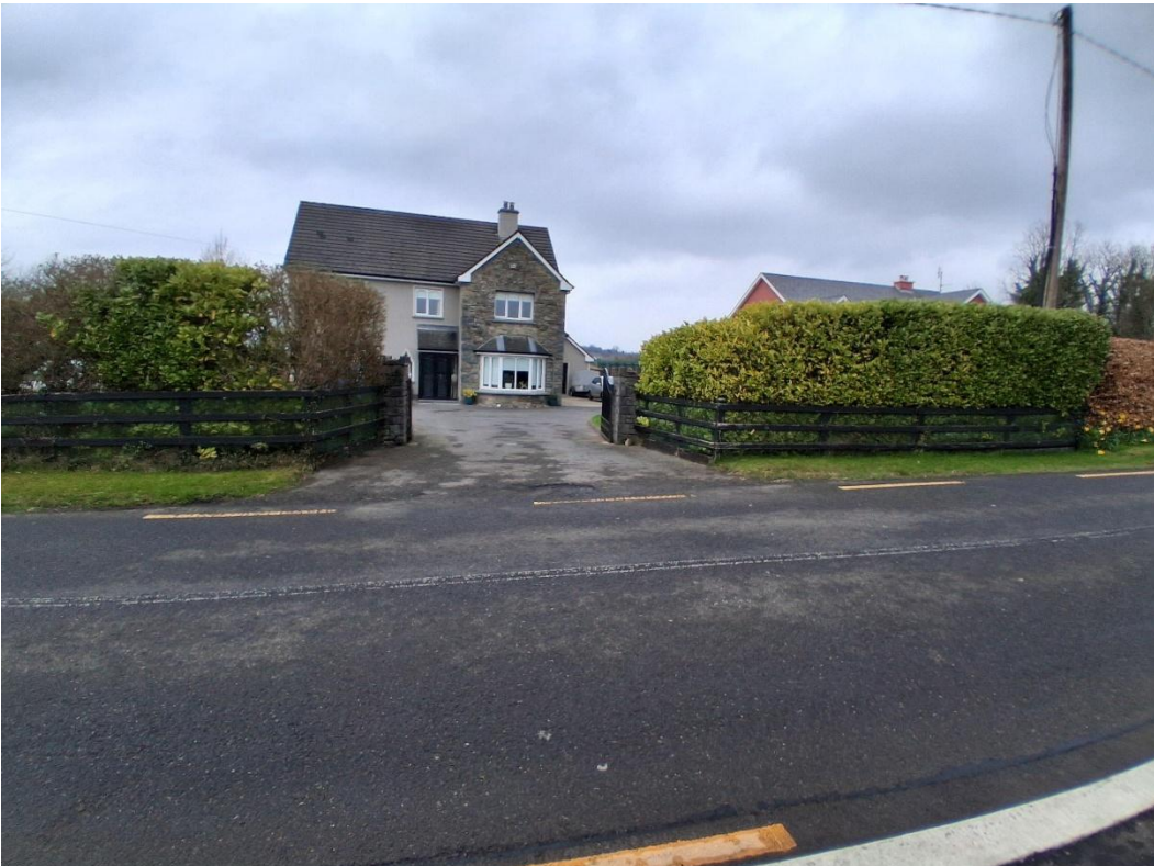
Fig. 2 Existing access serving adjacent dwelling
