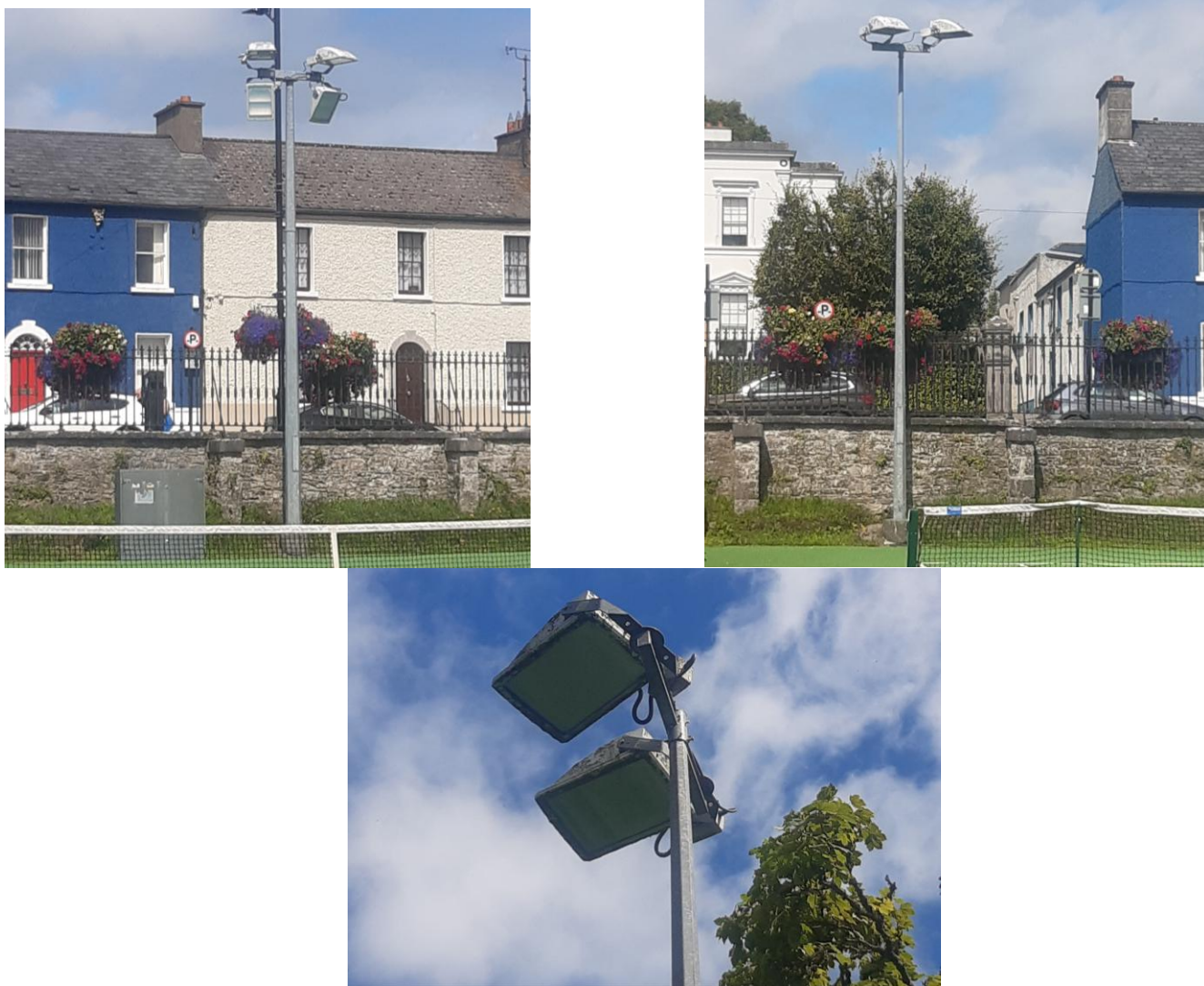
Fig. 1 – The existing 2 and 4 halide lamps and respective columns currently serving the tennis courts.
