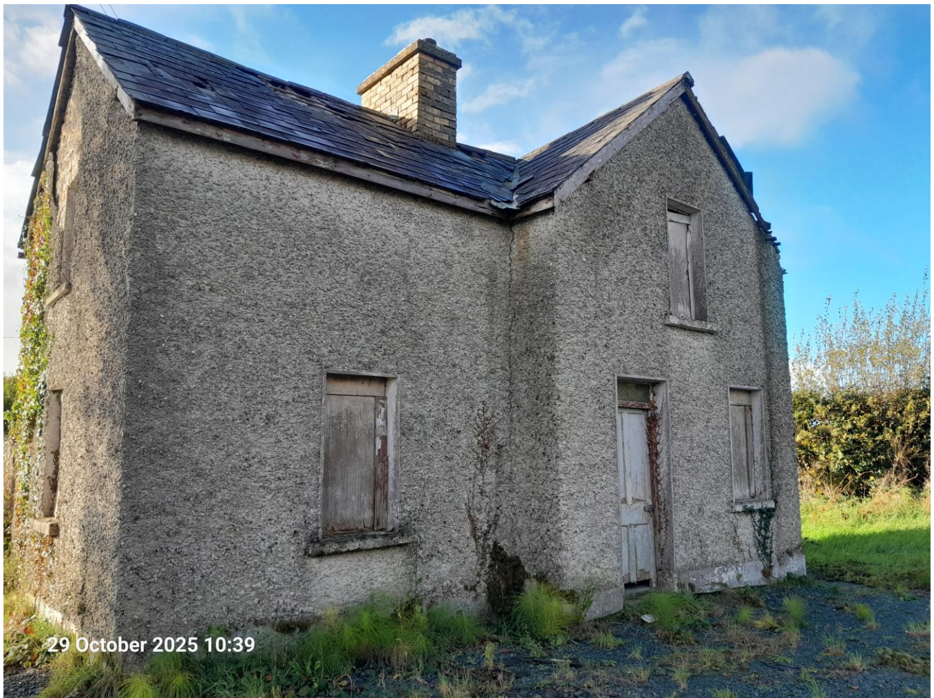
Fig. 1 – Subject derelict dwelling
