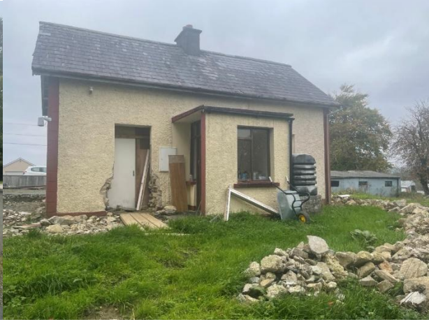
Fig. 2 This is the rear elevation
