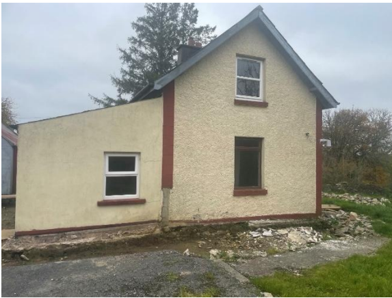
Fig. 3 The western elevation
