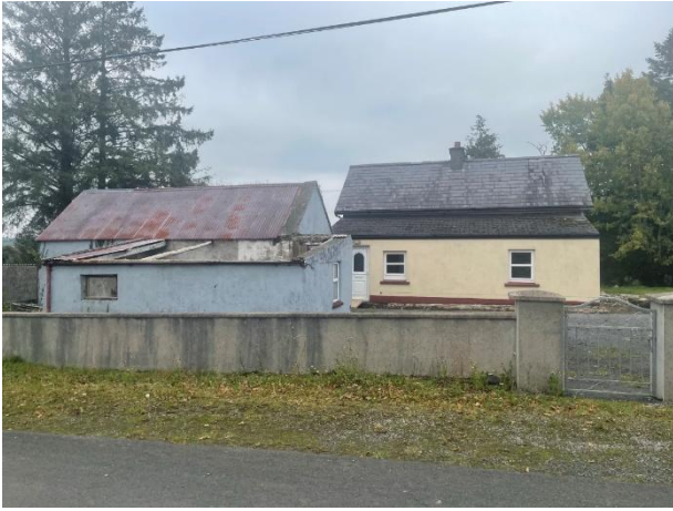
Fig. 1 The front elevation of the dwelling
