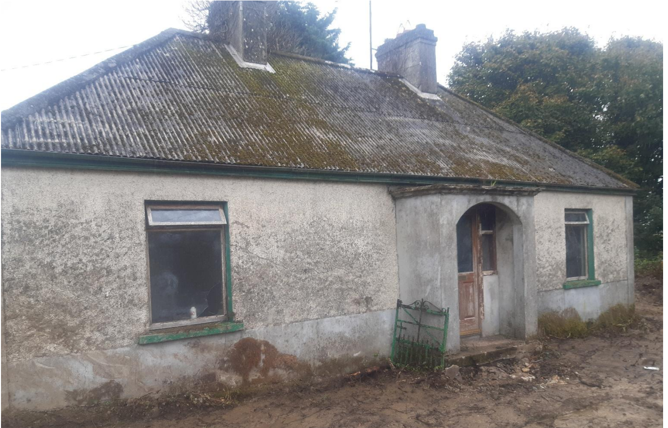
Fig. 1 The front elevation of the dwelling.
