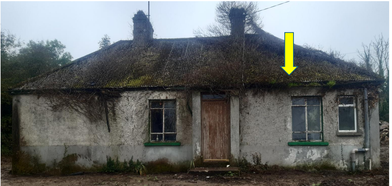
Fig. 2 This is the rear elevation onto which the applicant is proposing the 40m 2 extension.
