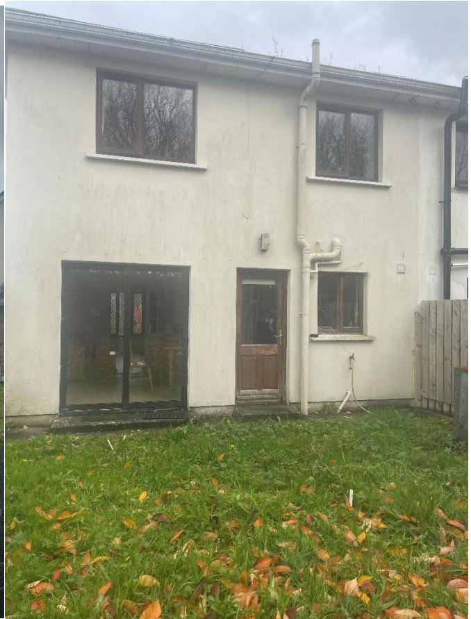
Fig. 2 This is the rear elevation
