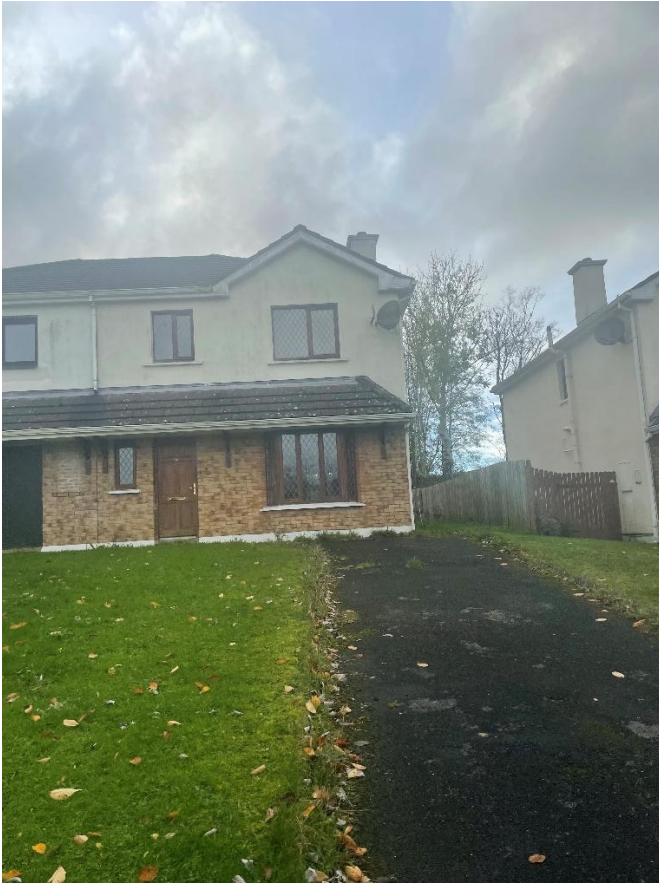
Fig. 1 The front elevation of the dwelling
