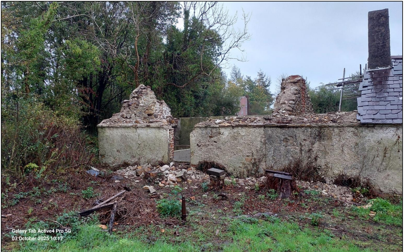
Fig. 5 – Remaining derelict section of single-storey rear extension (western elevation)
