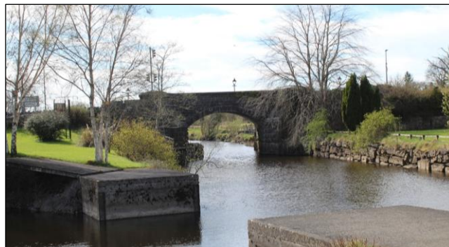
Photo of Leitrim Bridge in Winter 2025.
